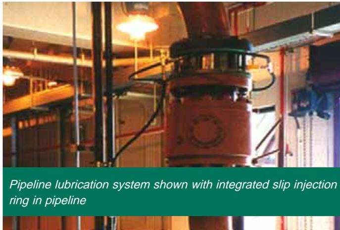
*Pipeline lubrication system shown with integrated slip injection ring in pipeline*
