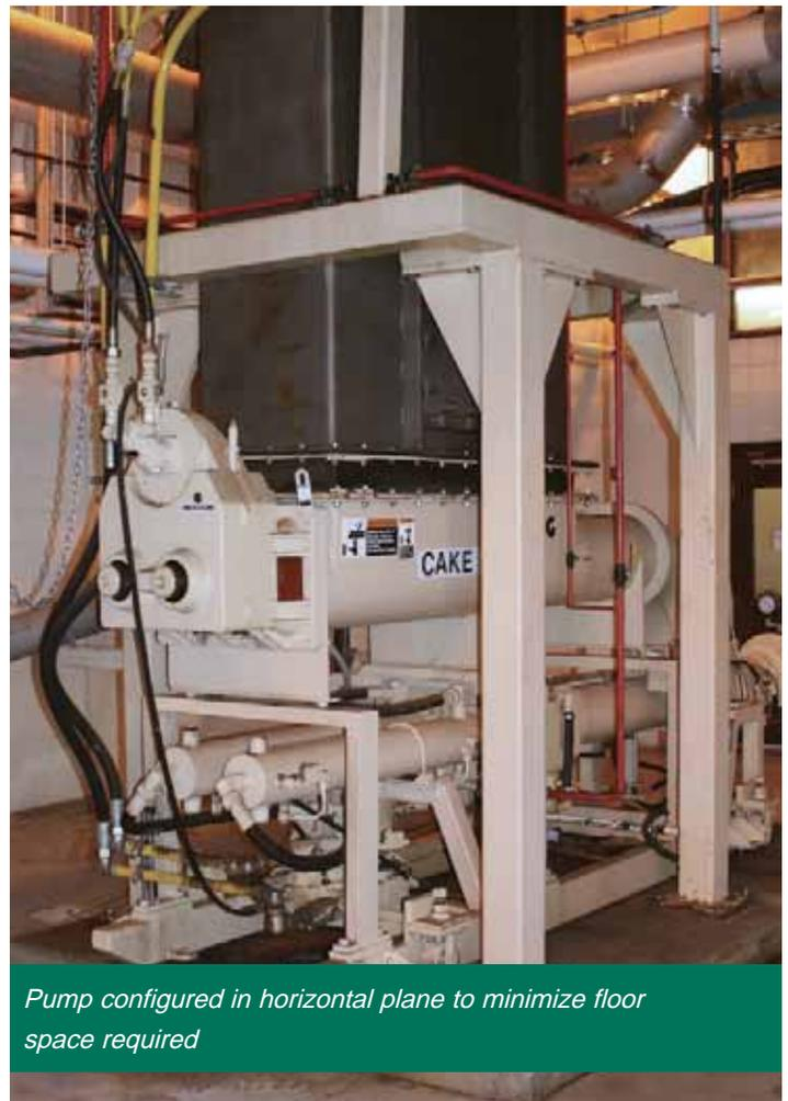
*Pump configured in horizontal plane to minimize floor space required*
