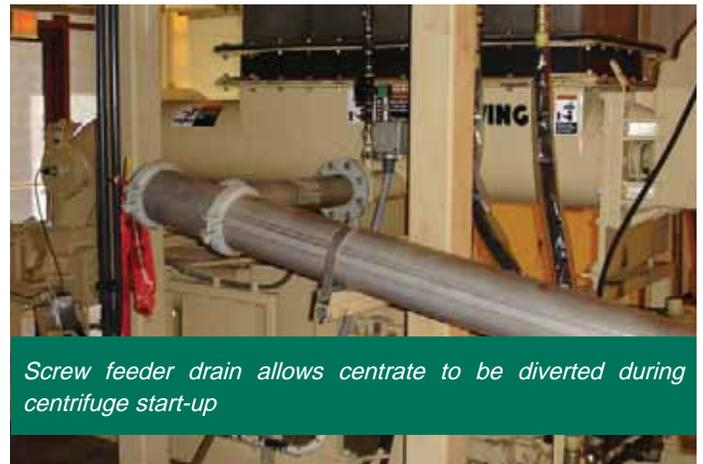
*Screw feeder drain allows centrate to be diverted during centrifuge start-up*
